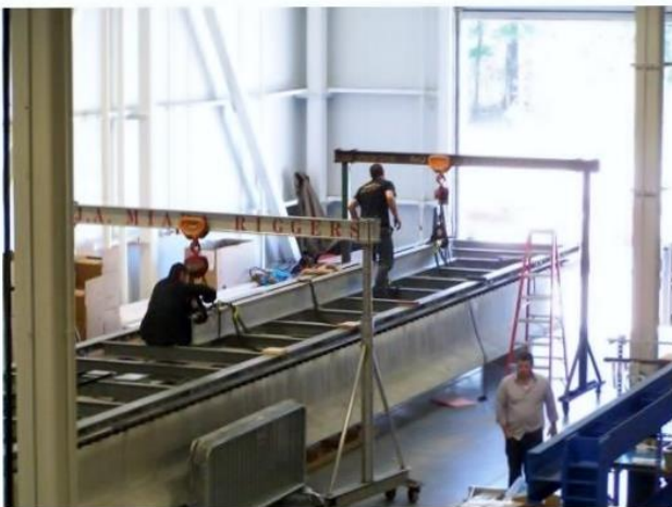
Figure 5a. Track structure being prepared for removal.
